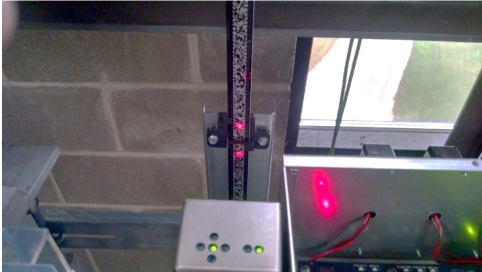
Figure 2-21: APS Selector Alignment Spotlights
