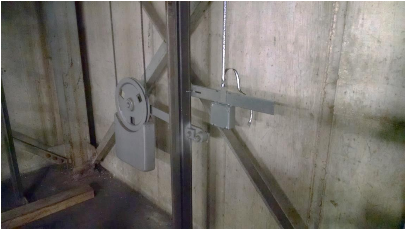
Figure 2-8: Encoded Tape Mounting – Bottom Bracket
