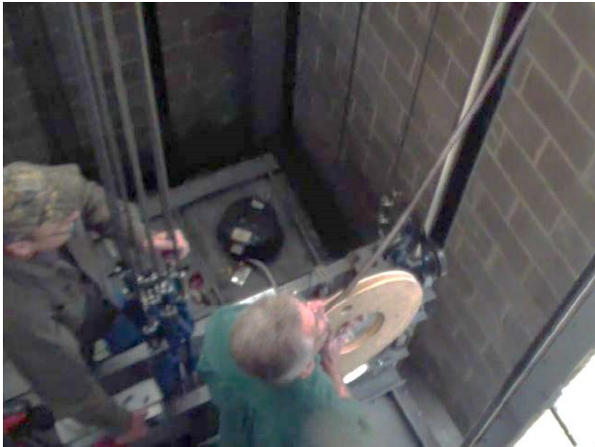
Figure 2-5: Unroll the Encoded Tape
